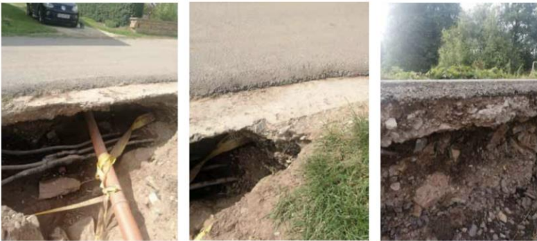
After heavy flooding the subbase is gone, the NovoCrete® base layer is still there!
