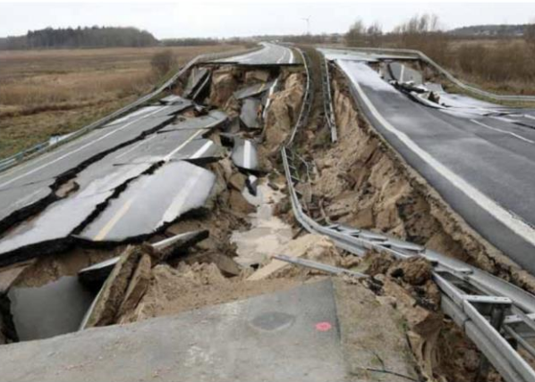
After heavy flooding the entire subbase and base layers are completely destroyed!
